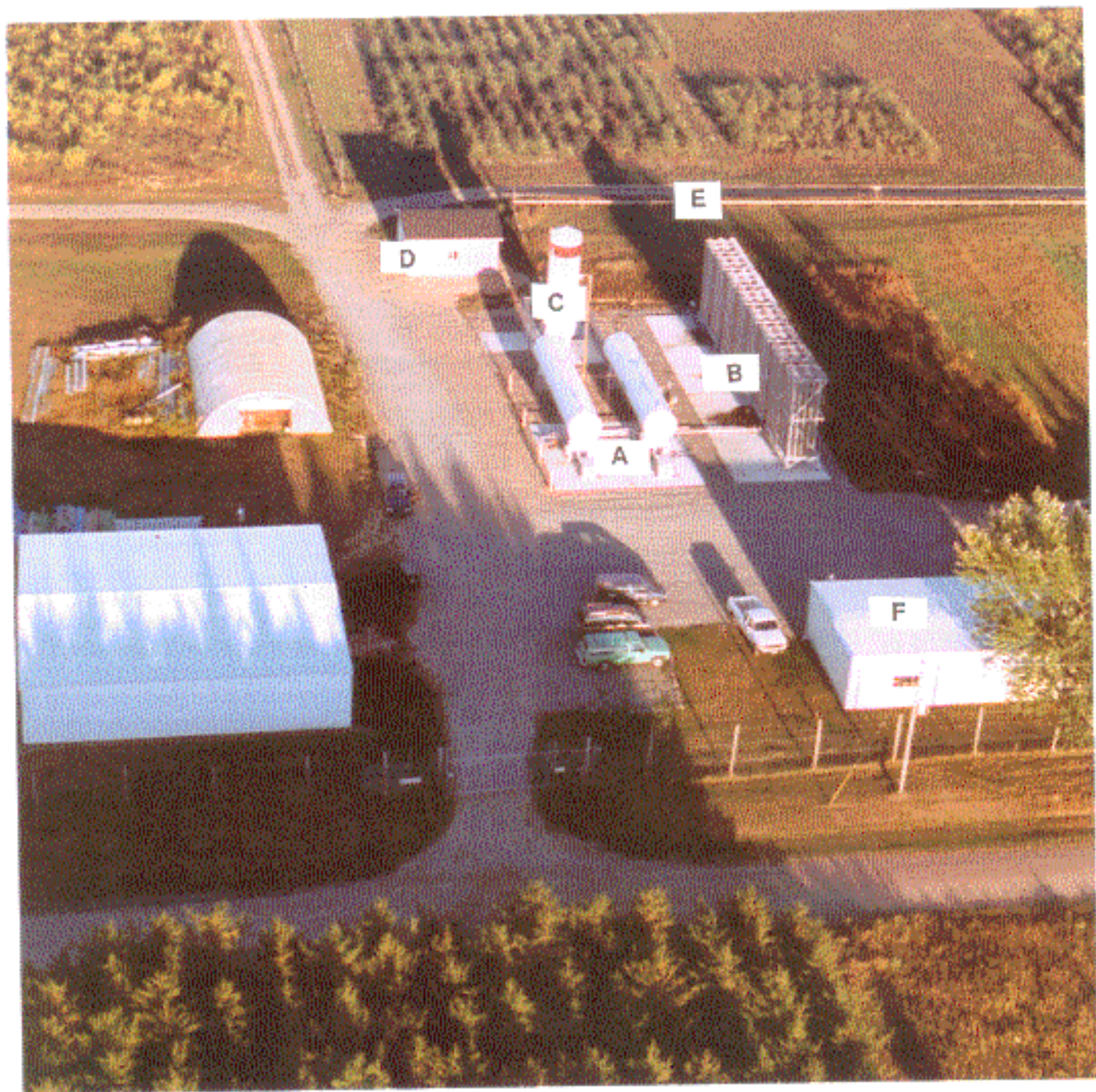
Figure 11.—Central control systems for \text{CO}_2 , liquid \text{O}_2 , \text{O}_3 production, and gas distribution. A. Liquid \text{CO}_2 storage tanks. B. Ambient-air heat exchangers. C. Liquid \text{O}_2 storage tank. D. Ozone generation building. E. Carbon dioxide and \text{O}_3 gas distribution lines. F. Main computer control building and shops.
